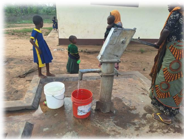
Wasser Handpumpe in Nyangao, 12.12.2024
